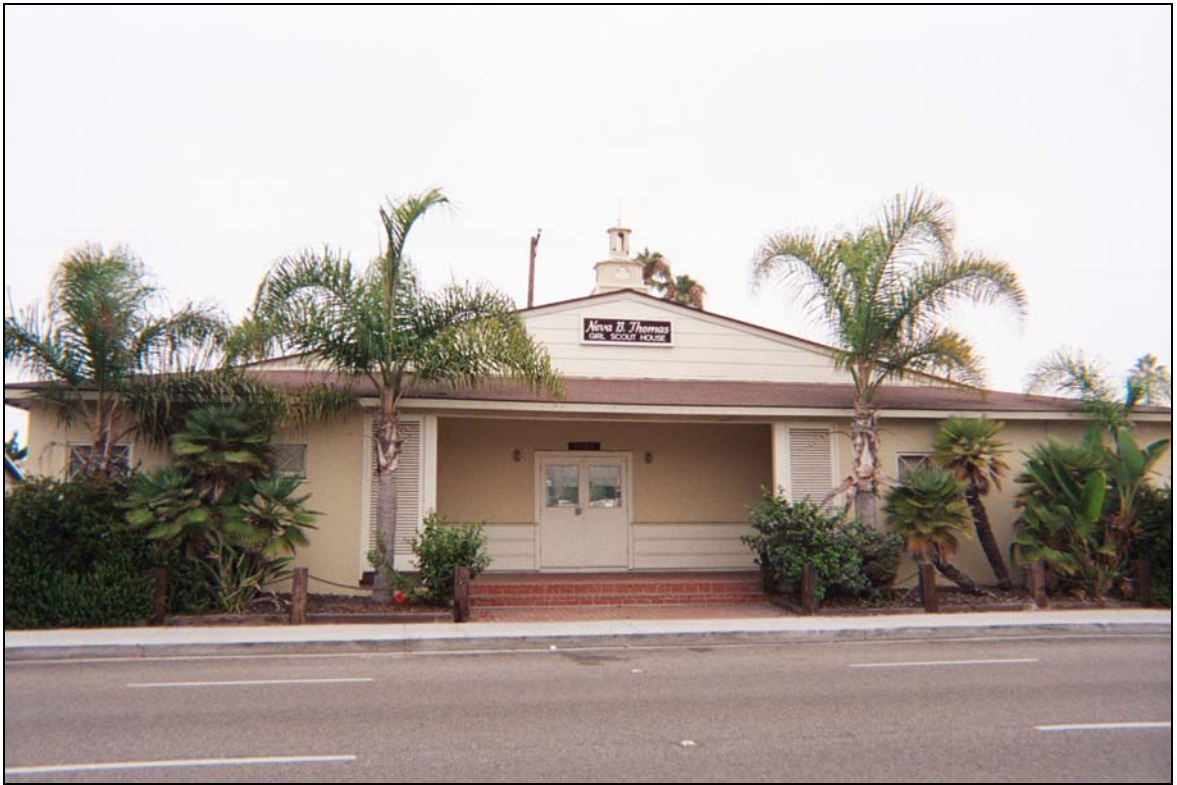
Photograph 11. View of the Neva B. Thomas Girl Scout Building, facing north.
