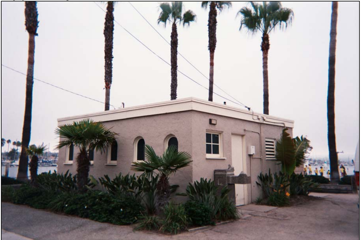
Photograph 8. View of the 19 th Street Restroom, facing northeast.
