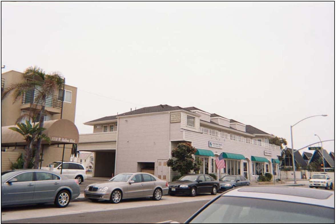
Photograph 13. View of off-site 1510 West Balboa Boulevard and the Associated Reality Building, facing northeast.
