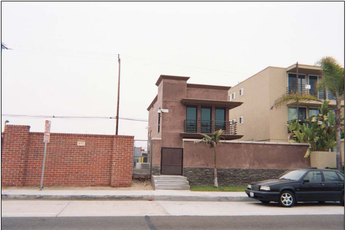
Photograph 14. View of the off-site Southern California Edison Property, facing north.
